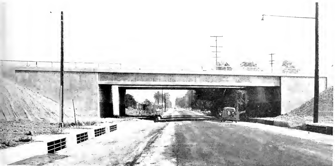
Looking southerly along San Antonio Avenue showing dual Ramona Freeway bridges
